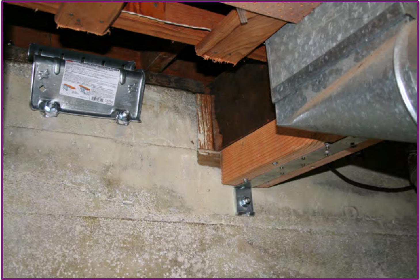
Post & beam reinforcement.
