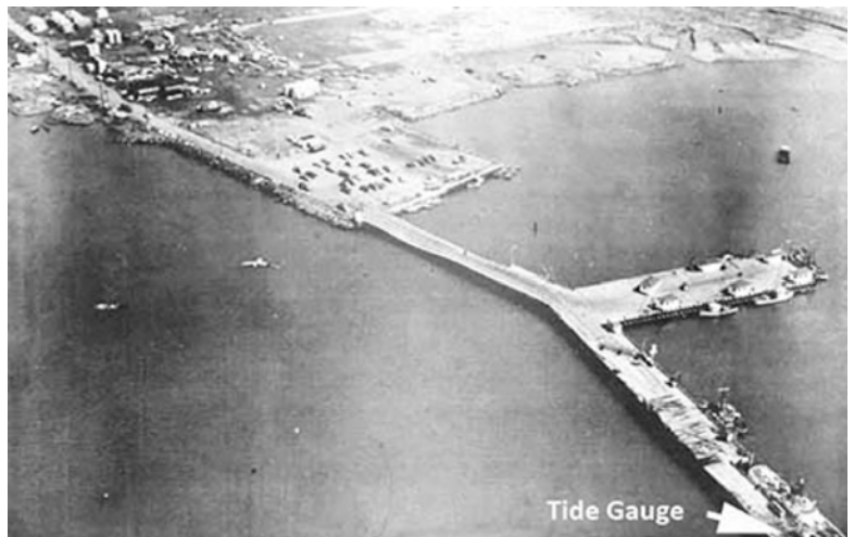
Figure 16. Citizens Dock on April 1, 1964 after the tsunami. The tide gauge was located near the end of the badly damaged Lumber Dock.
