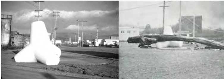
Figure 14. The tetrapod at the corner of N and Front Street was displaced about 3.5 meters in the 1964 tsunami. The photo of the right was taken the day after the tsunami and shows the culprit – the log whose impact provided the necessary force to move the 25-ton object.
